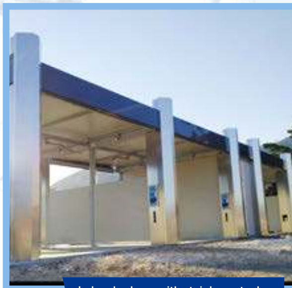
Labrador bays with stainless steel column covers - recessed lance holder detail.
