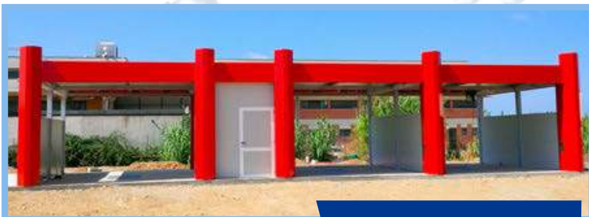
Labrador bays with painted column covers.
